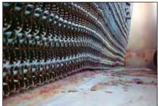
Other Manufacturer's – Hanging Sheets Extend to the Basin Floor "Difficult to Clean" Basin Floor
