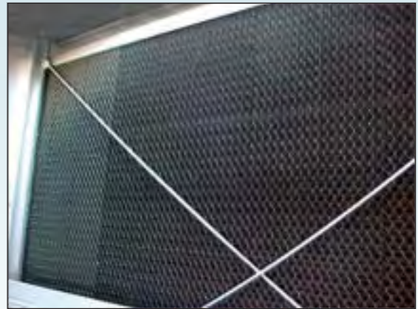
EVAPCO – Tightly Packed Eliminator Bundles
